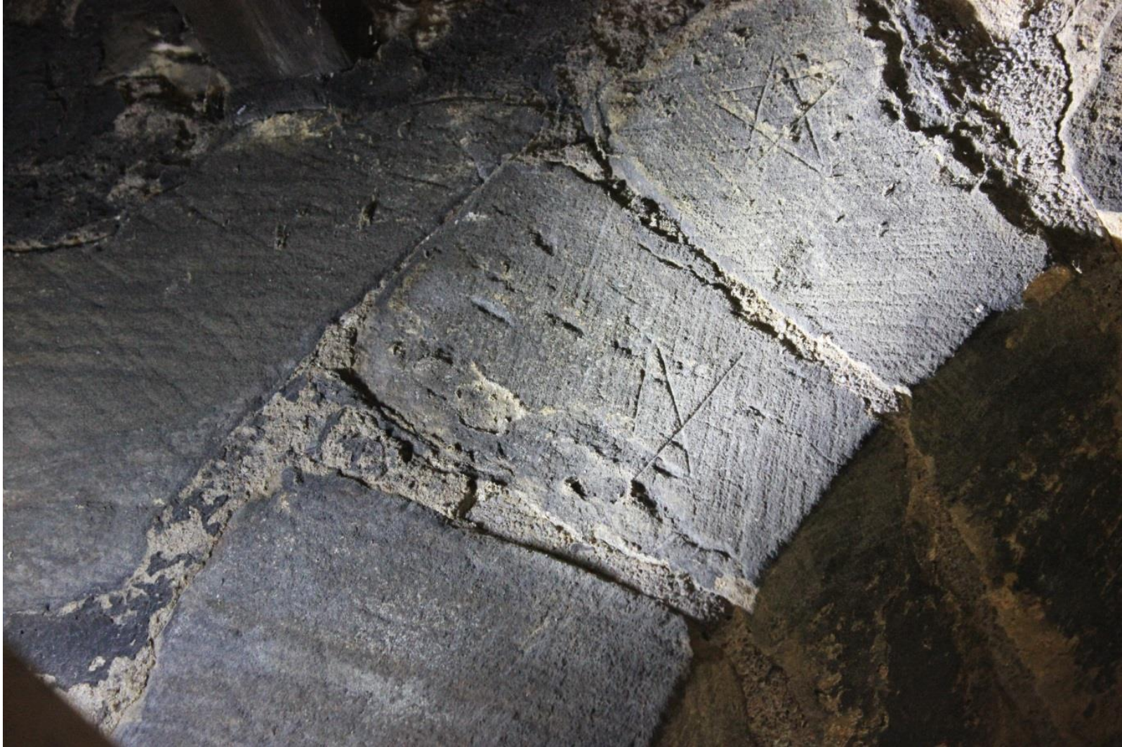
Mason 29 – Marks 715, 716 on the voussoirs of a window.
