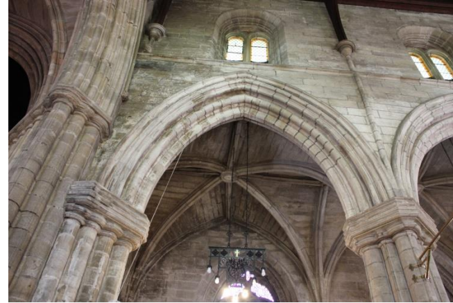
Upper wall of East Church Chancel
