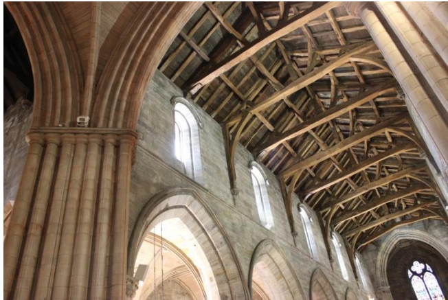
Upper wall of West Church nave
