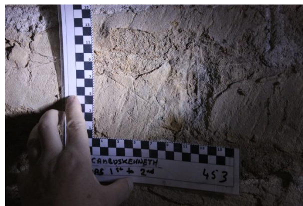
Mason 46- Mark record 0453 with spalling of stone
